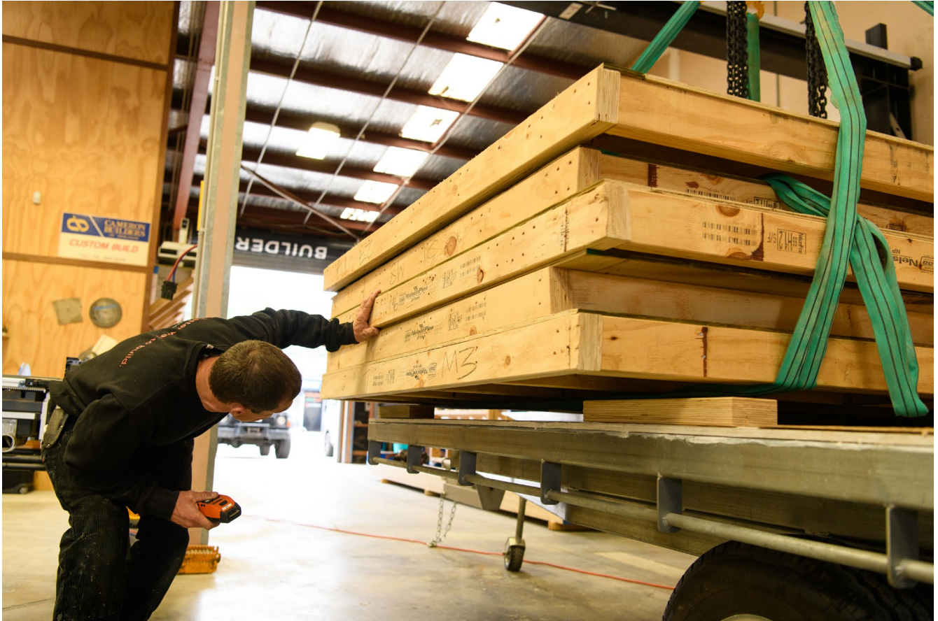
Ingo True loading finished prefabricated panels to a trailer.
