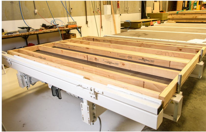
A prefabricated panel being built at Frankhouse.
